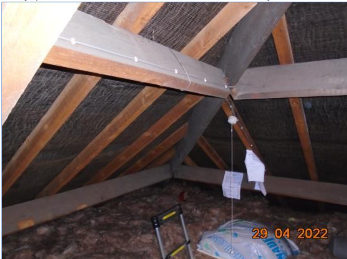
Photograph 6 – Internal view of the roof structure of the main dwelling.
