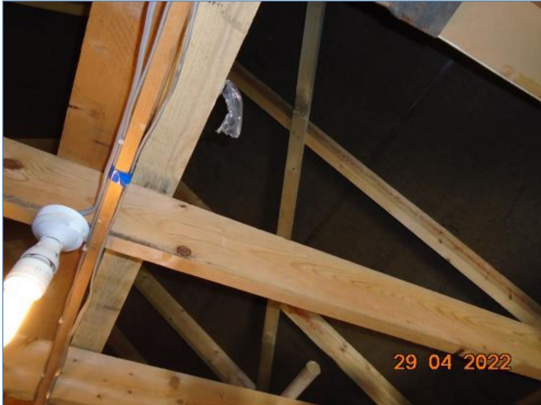
Photograph 7 – Internal view of the roof structure of the detached garage.
