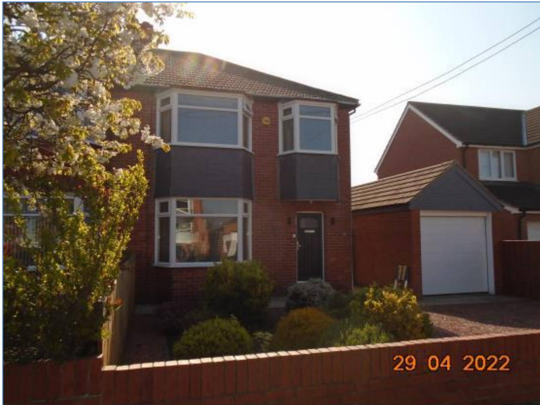
Photograph 1 – Front (north-west) elevation of the property.
