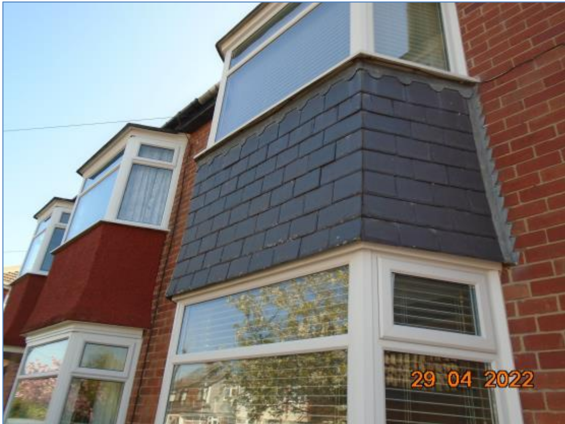
Photograph 5 – Close fitting slate hanging tiles on the front elevation.
